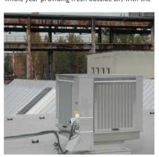
cooling function only being operated when conditions dictate. At the same time the hot air inside the building is normally removed at high level by natural or mechanical ventilators, providing a pleasant temperature at working level.
