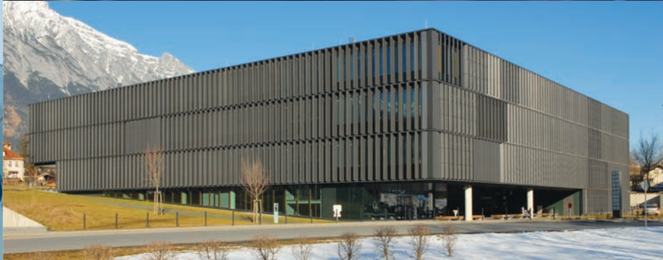
Tilak Competence Centre, Innsbruck, Austria. 964 moveable louvers comprising an area of 2925m 2 of solar shaded façade.
