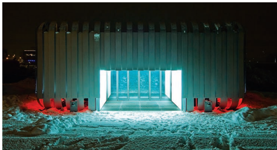
iHomeLab, Switzerland. The louvers give an appearance of a fish moving. The louvers themselves consist of a total of 380 fixed and 300 moveable louvers installed vertically on a building which has an exceptionally high thermal performance.
