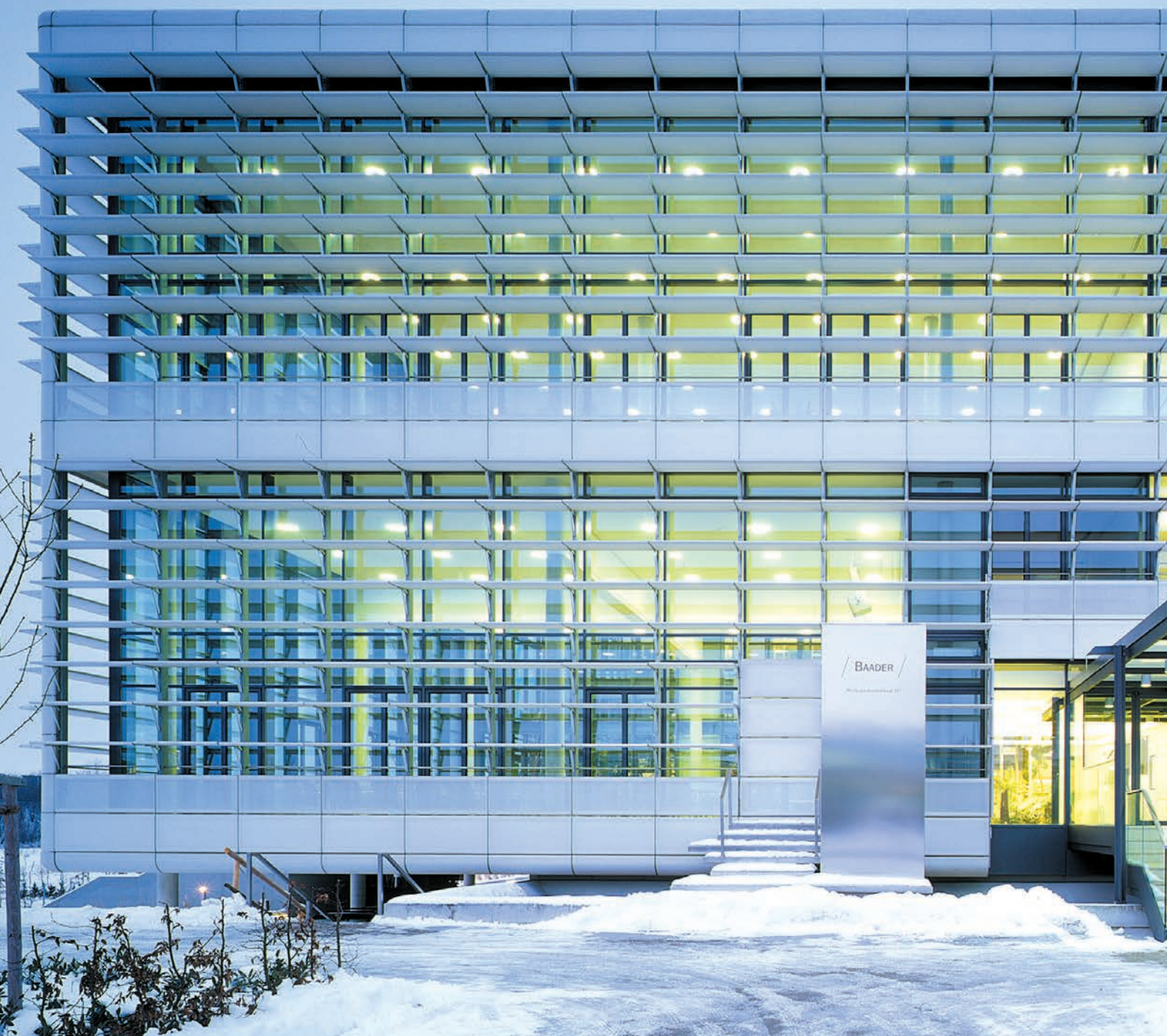
Baader Securities Bank, Munich, Germany. The building has been nearly entirely wrapped in louvers made of PTFE glass fibre Shadotex textile louvers. Louvres are individually adjustable and have greatly reduced the energy use of the building.
